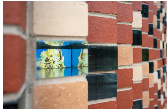
The Digital Bricks at the entrance to Science Gallery Melbourne. (photo: Toby Welch/Arup, 2021)
